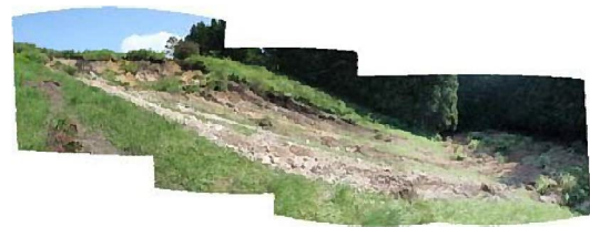
Landslide in the Yamaguchi Prefecture.
